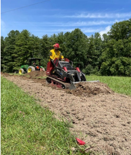
A DSRF ranger prepares the trail surface before the application of gravel to the new connector trail.
