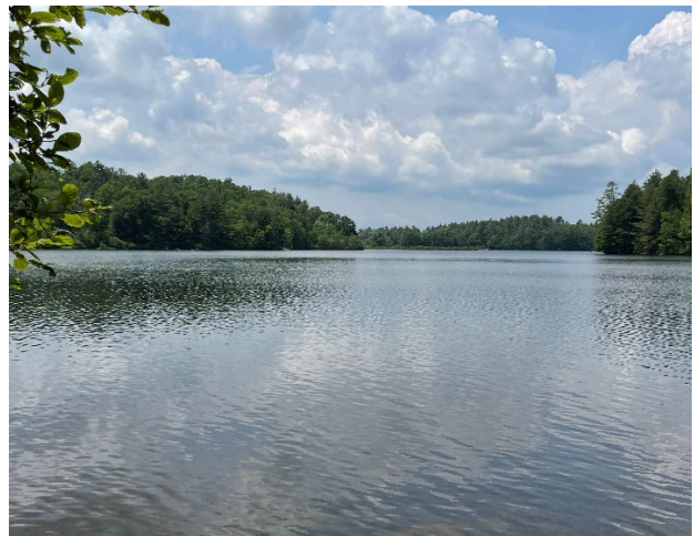
The Lake Julia dam has never been repaired or improved since its original construction in the late 1960s.
