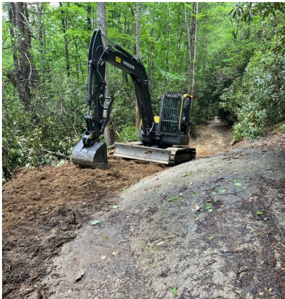
A DSRF ranger repairs severe erosion on Lake Imaging Road.
