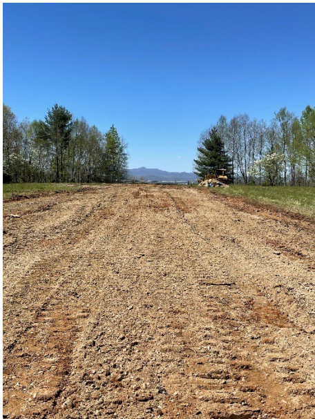
The airstrip after the removal of a section of asphalt.
