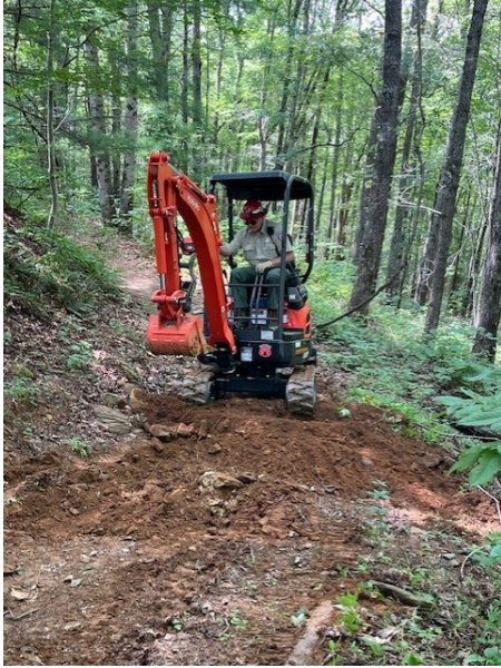
A DSRF ranger uses the grant funded mini excavator to perform work on a narrow multiuse trail.
