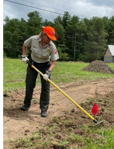
A DSRF ranger uses hand tools to clear debris from the prepared trail bed and adjacent meadow.
