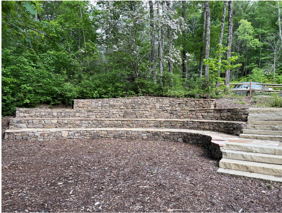
Figure 4: The amphitheater constructed at the visitor center during FY23-24.
