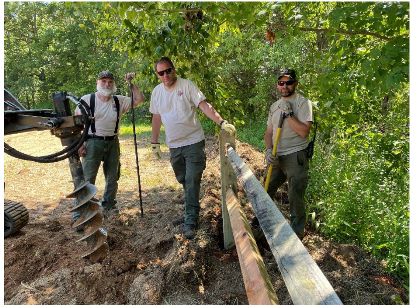
DSRF rangers installing fencing at the end of the airstrip.
