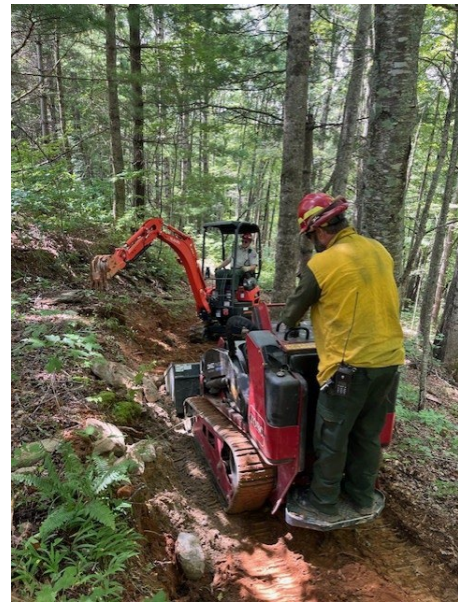
Two DSRF rangers use machines designed for narrow locations to work on trail.
