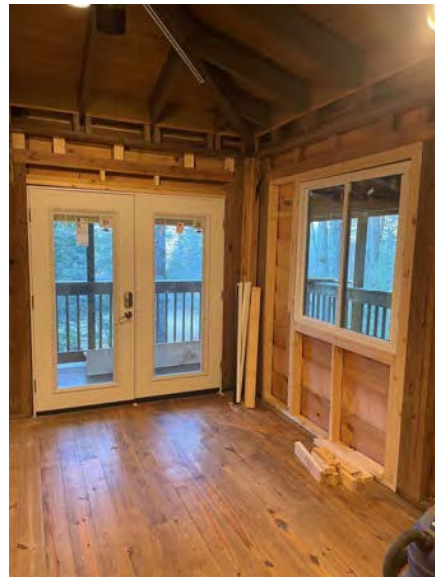
HESF Forestry Center interior during renovation.
